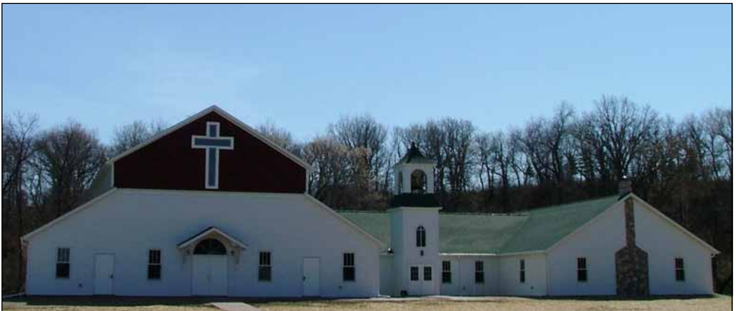
The Park River Bible Camp Chapel as it now stands completely renovated.
