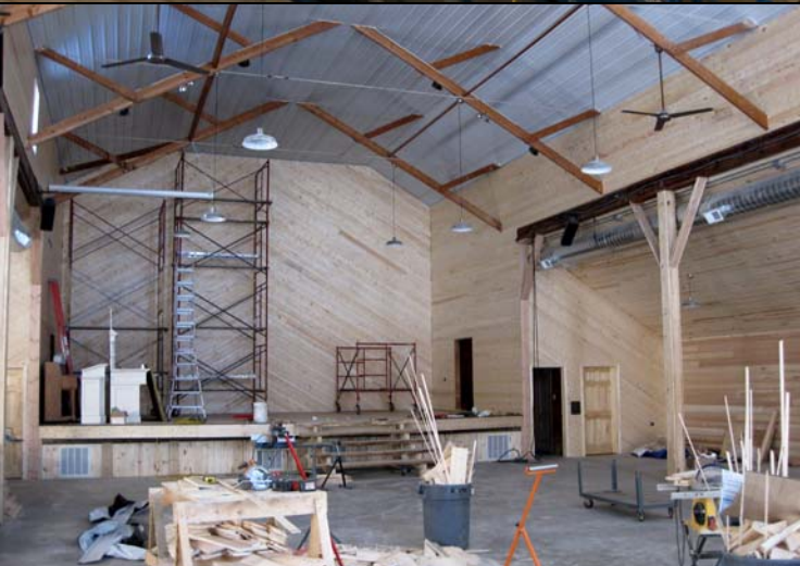
Top: Two volunteers finish siding the rear wall of the Chapel.
