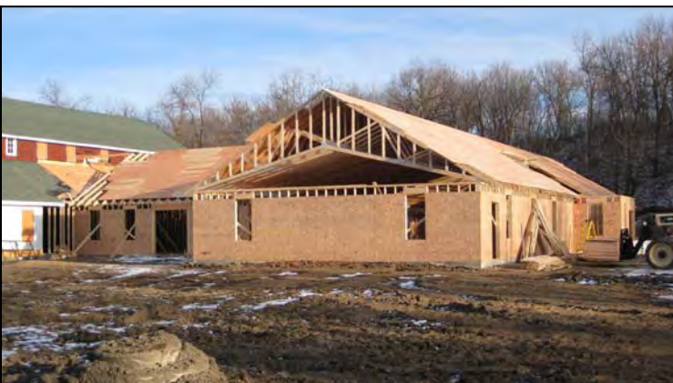
Much of the framing for the addition has been completed.
